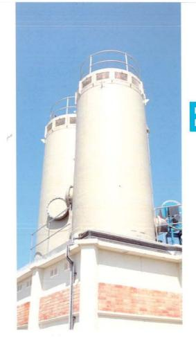
Forbes Degassers are well proven as an efficient, reliable and cost-effective approach to reducing the problem of dissolved CO, during water treatment.
